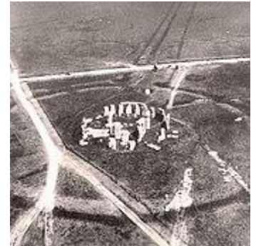
Stonehenge from the air. Taken by 2nd Lt Philip Henry Sharpe in Summer 1906 from a Royal Engineers' tethered balloon.
